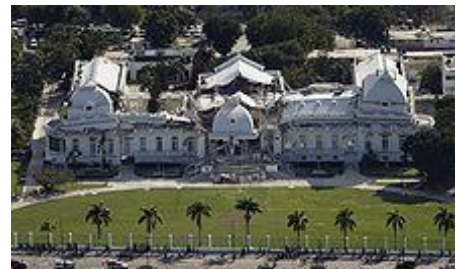
Day 1 - Collapse of the Presidential Palace
